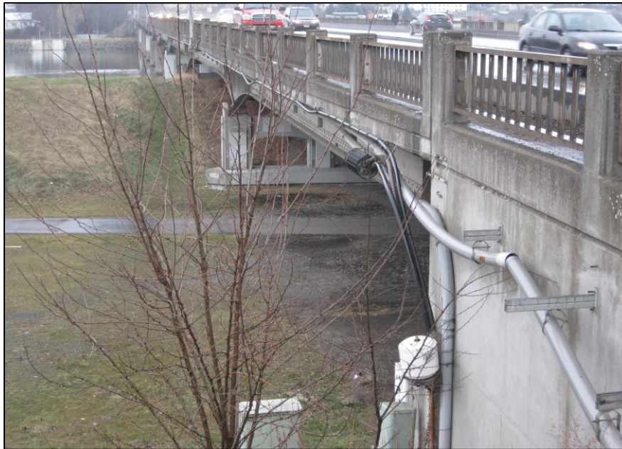
Figure 8: View from the north abutment of the utility attachments to the east side of the bridge
