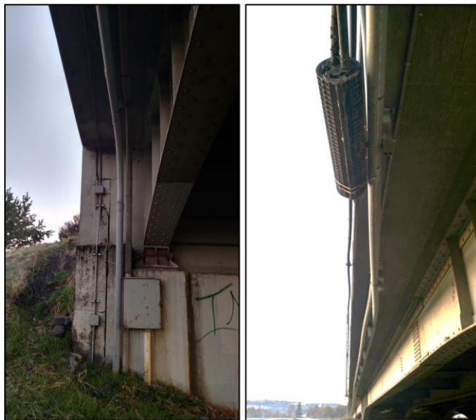
Figure 7: Utility hangers of the (a) west and (b) east sides of Abutment No. 2 on the north end of the bridge
